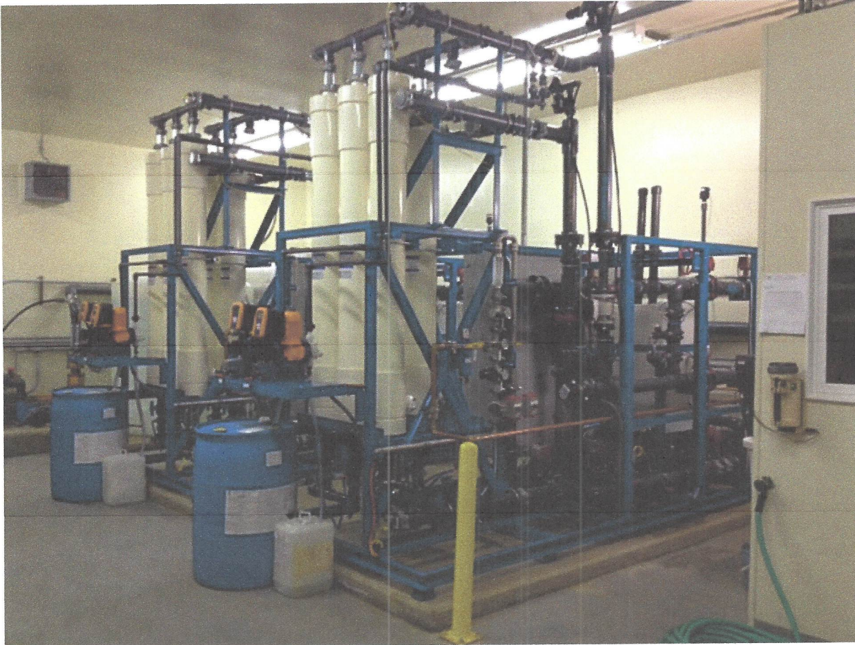
Water Plant Membrane Skids
